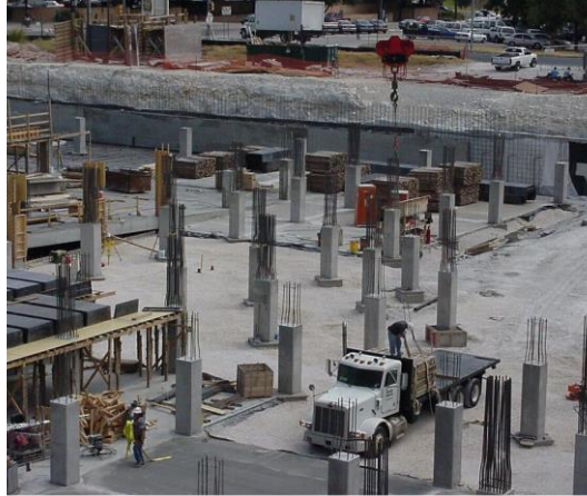
Columns and bearing walls
