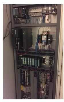
New Control System was installed using Siemens Sinamics Drives and S7-400 PLC's. This Control System upgrade simplified the Pinch Roll project integration at the Florham Park facility.
